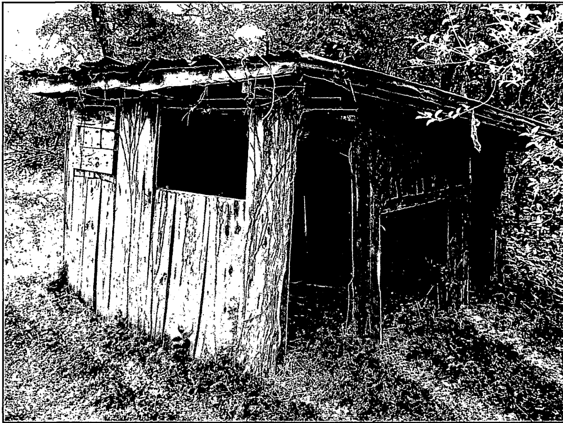
Figure 20. HR-4, animal shelter, looking northeast.
