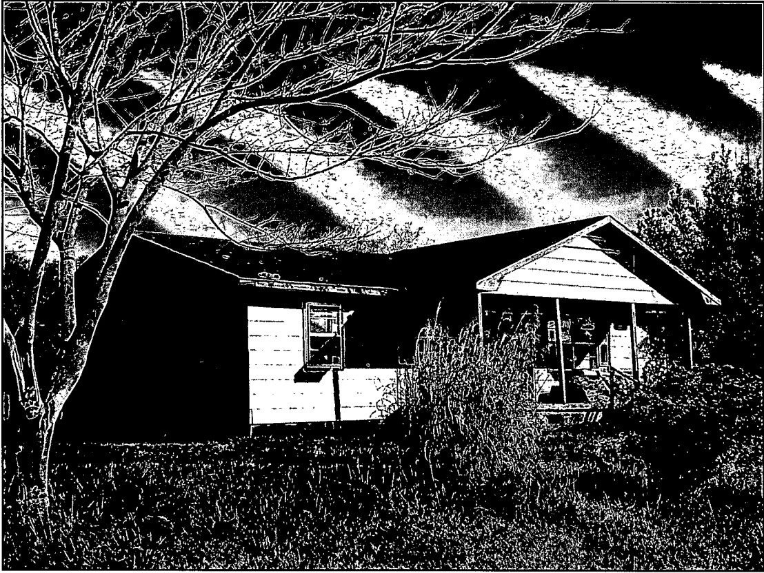
Figure 21. HR-5, façade and side elevation, looking northwest.
