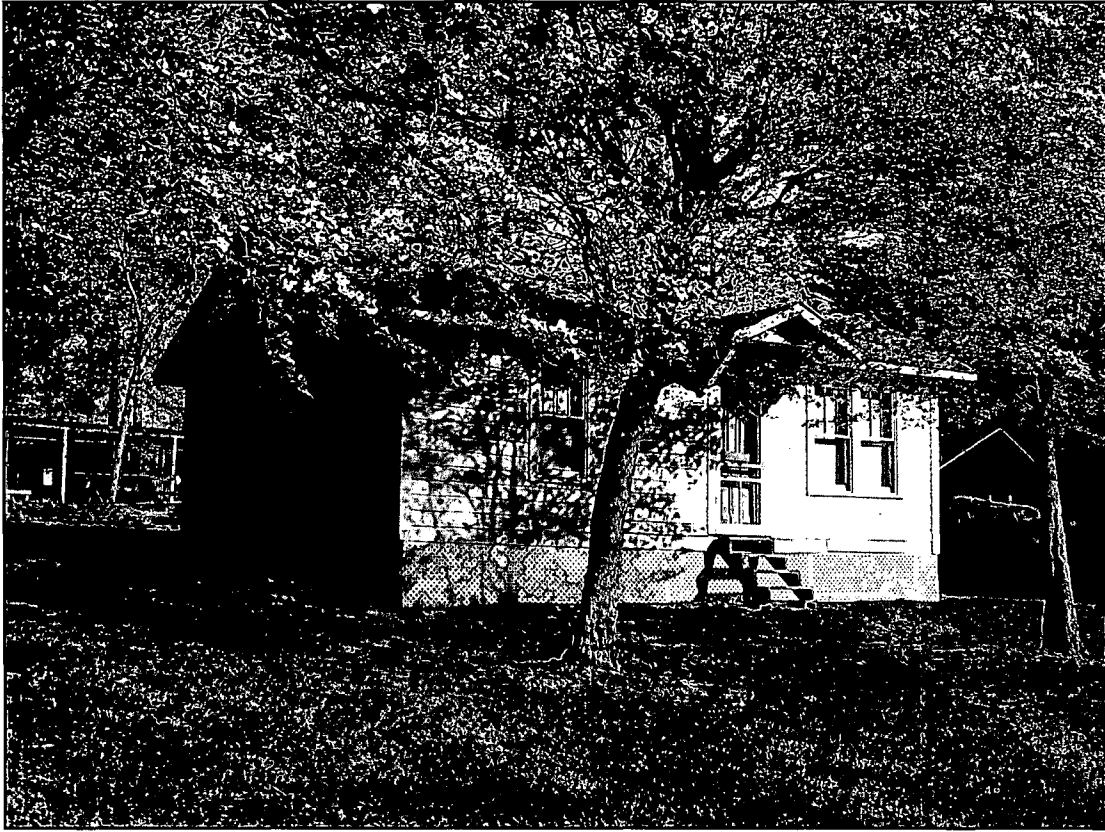
Figure 7. HR-2, Creekside Historic District, 1952 summer house, looking northwest.
