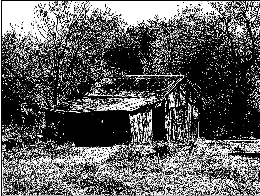
Figure 10. HR-3, barn, looking southeast.
